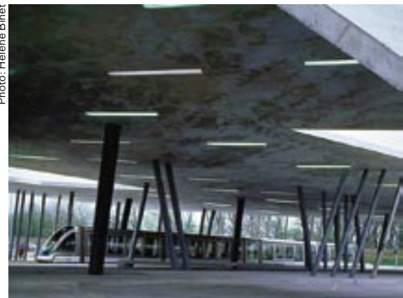
Car park and terminus building, Hoenheim Nord, Strasbourg, France. Architect: Zaha Hadid. Award won: European Union Prize for Contemporary Architecture – Mies van der Rohe Award 2003.
