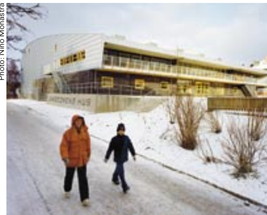
Young People's Building in Rinkeby, a multi-cultural suburb to Stockholm, Sweden. Architects: Anders Bergcrantz, Bergcrantz Arkitekter AB. Nominated to the Kasper Salin prize 1999.
